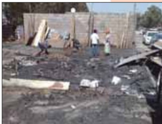
40 shacks destroyed. Sizwe is rebuilding his shack where it once stood. The fire started in the shack that was located where the two people are standing. In the background is the spaza shop fire wall.
